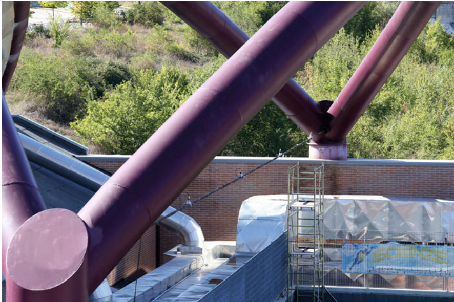
Fig. 6.25 Installation of the prototype of monitoring system on one of the cables of a sample steel arch
